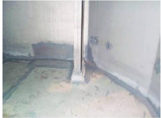
**RESULT:** The BIO-DUR 561 coating was applied by university personnel to selected portions of the aluminum liner including weld seams along the pool floor, around beam flanges, and on several areas of pitting.
