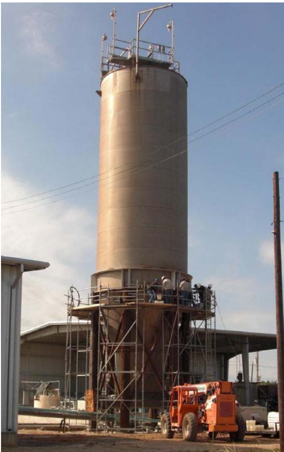
Elevated silo with pumping in progress
