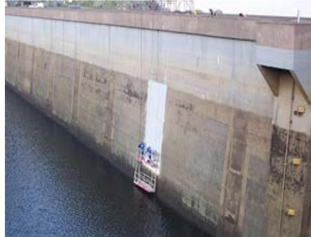
employed in the full-scale coating. The two-tiered scaffold shown was used to provide close and safe access to the dam face.
