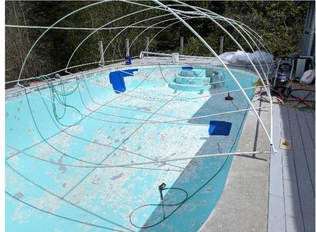
The image above shows the pool after initial preparation of the aged coating. The photo below is the transformed pool after FASTONITE 700 application.
