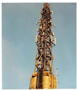
**THE SOLUTION** TOWER-GARD 568 was especially formulated to provide a solution in which single heavy coating, tolerant of compromised surface preparation, would provide good long-term protection to bare steel, previously painted surfaces and worn galvanized surfaces.
